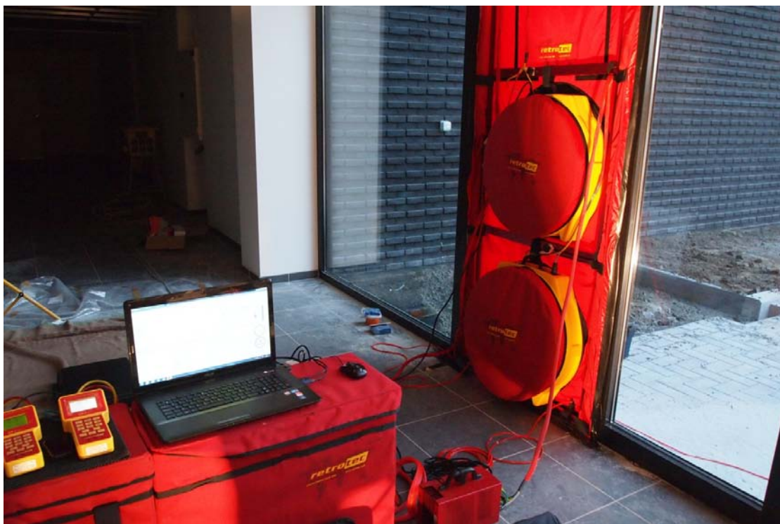
Figure 2 - Blowerdoor meting | EPB LIPA BVBA
